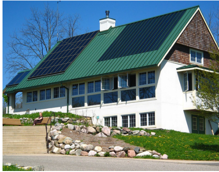
Figure 18: A house with two-fold roof with integrated solar modules on the south side [10]
