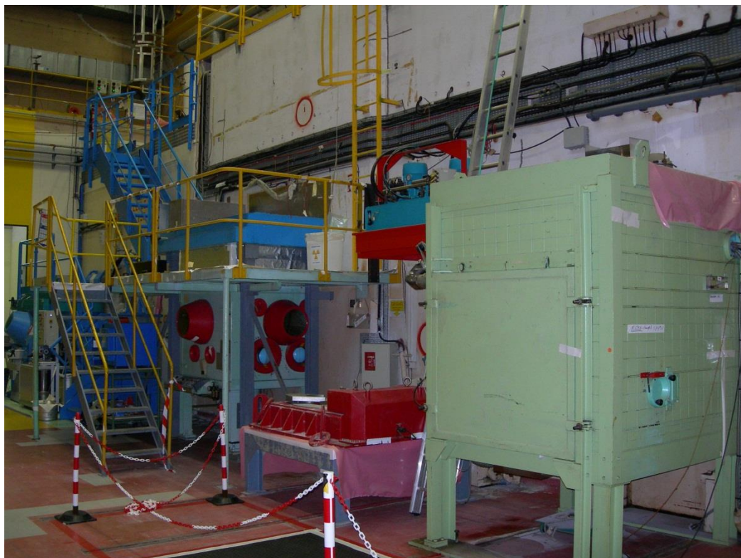
Building 120 - Backward area
