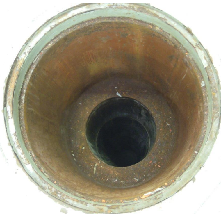
Building 114 - The open pit
