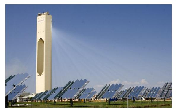
Figure 3 – Solar power tower
