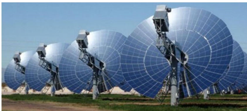
Figure 2.6: Parabolic dish heliostats with point receivers [21]
