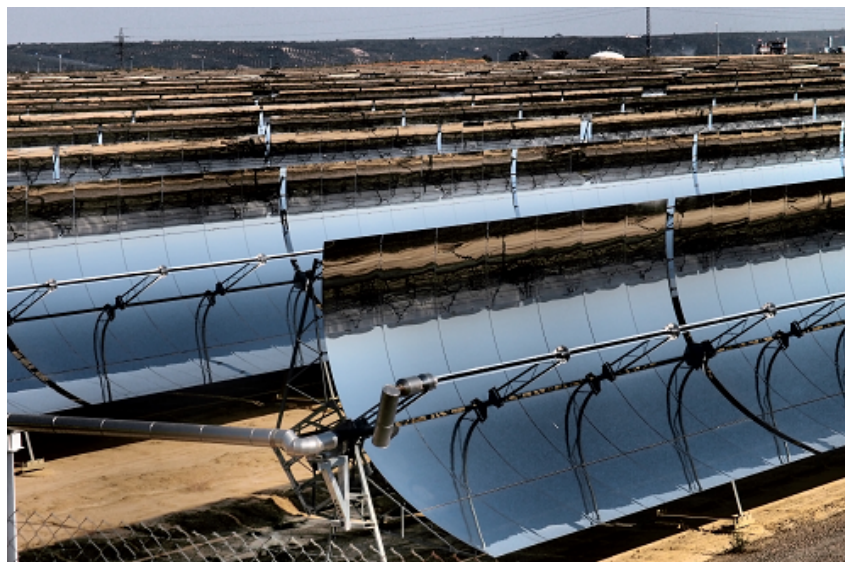
Figure 2.5: Parabolic trough mirror with linear focus receiver [14]
