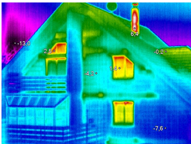
Fig.7.: The measurement of the facade temperature profile.
