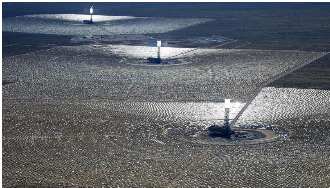
Obr. 6.2 Ivanpah Solar Power Facility
