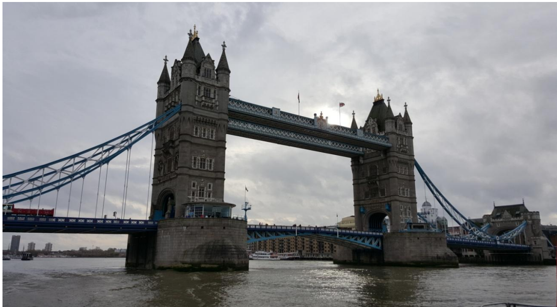
Figure 1 Tower Bridge (Dominik Novák's Archive)
