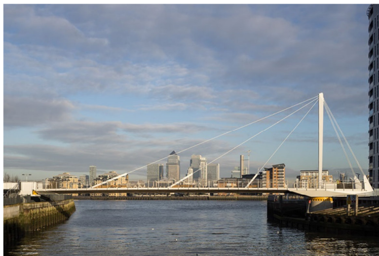
Obrázek 1.20: Otočný most Greenwich Reach [Zdroj: https://eadonconsulting.co.uk/project/greenwich-reach-swing-bridge/ ]
