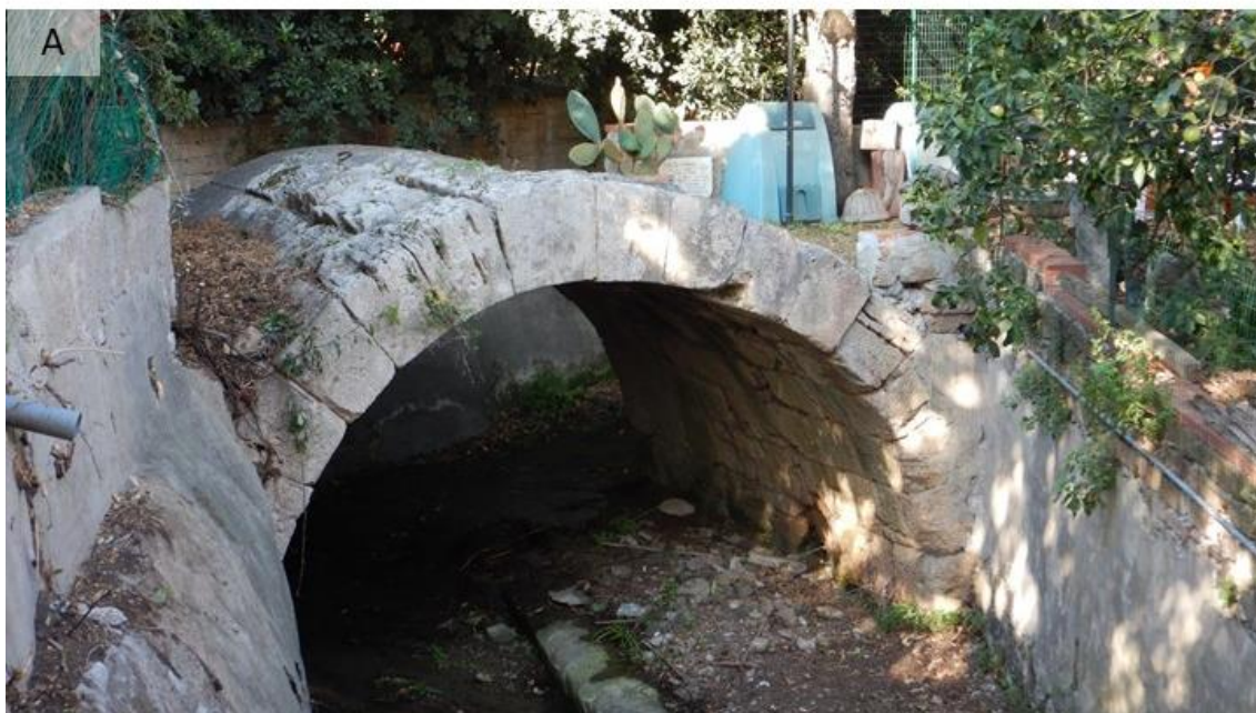
Fig. 150 A: the bridge in 2019.
