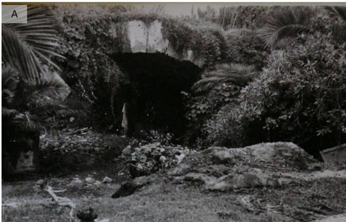
Fig. 181: the bridge on the documentation of SAEM.
