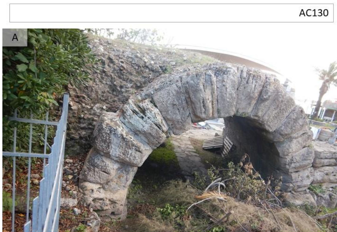
Fig. 148 A: the state of the bridge in 2019.
