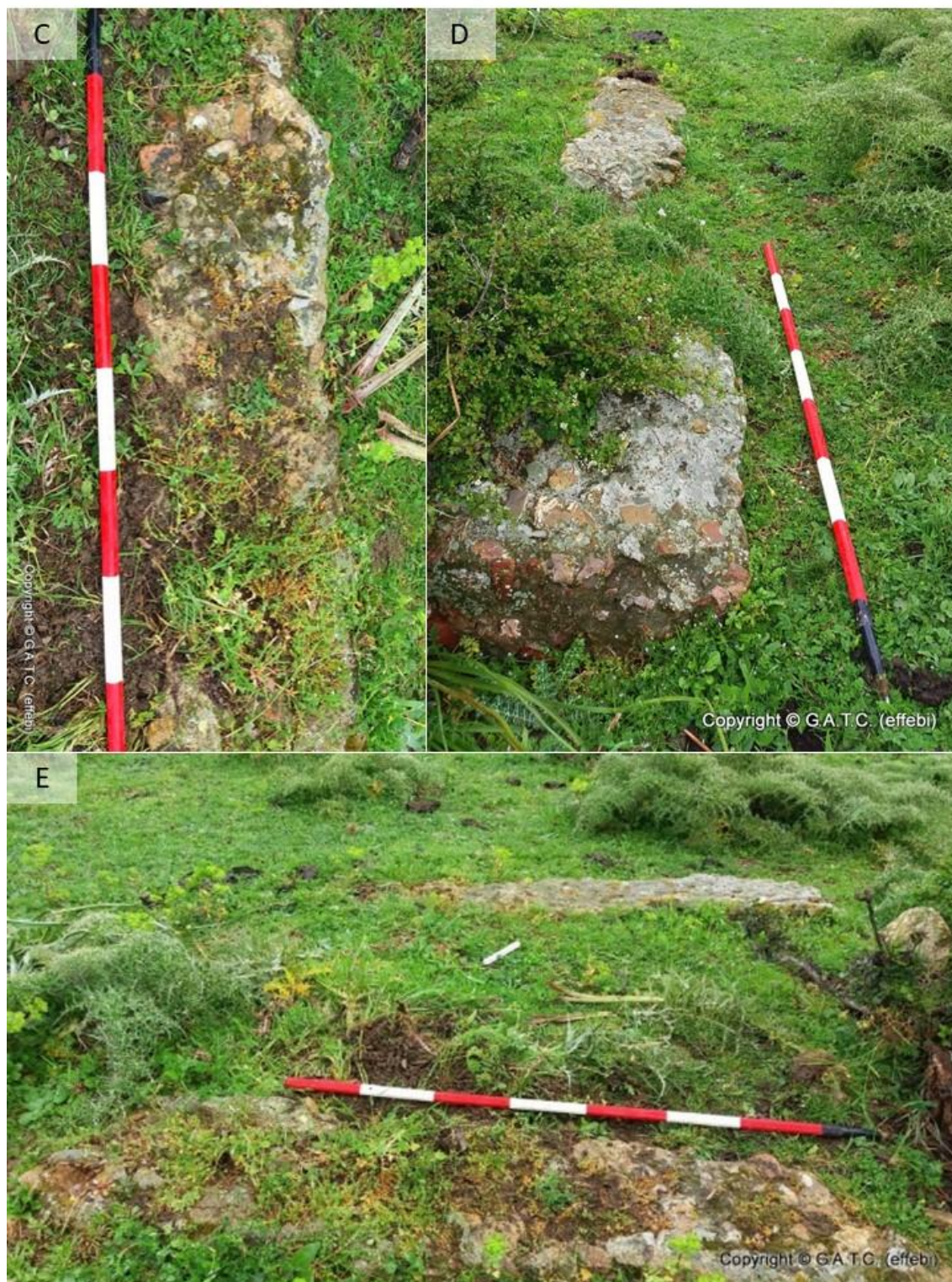
Fig. 129 C, D, E, details of walls relicts (from the archive of Bruno Fantozzi).
