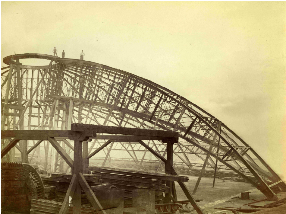
Picture 21: Construction of the roof
