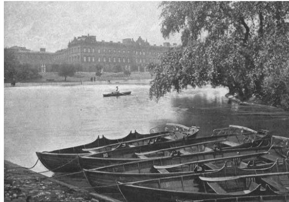
Picture 29: Buckingham Palace in 1896, seen from St. James's Park
