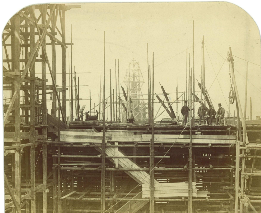
Picture 20: Construction of the Hall between 1867 and 1870
