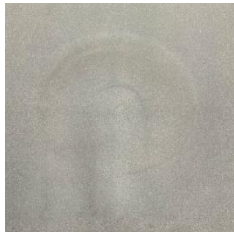
Fig. 4. Picture of the damages left to the surface after the test (the photo has been treated to enhance the effect, otherwise inappreciable).
