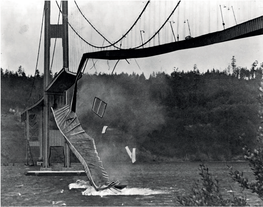
Figure 1.1: Tacoma Narrows Bridge collapse on November 7, 1940. Retrieved from [24].
