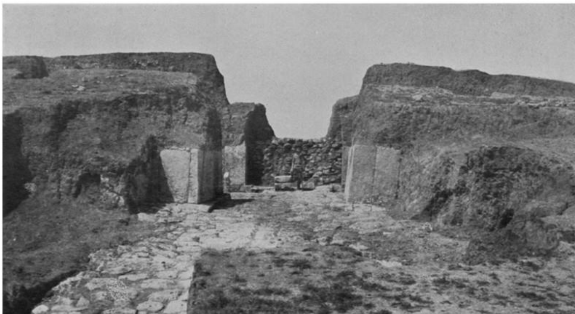
FIG. 5.—GATE 7, FROM WITHIN THE CITY
